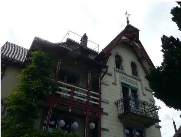
Friedheim, Detail Obergeschoss. [Foto MEC 2014]
