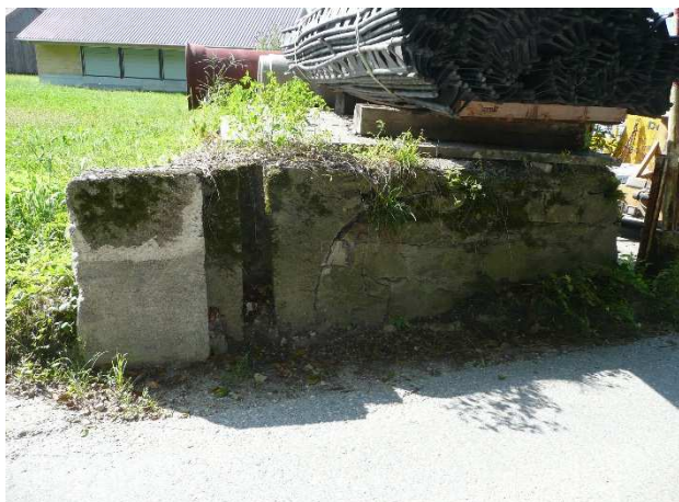
Mauer Wilertobel, Details. [Foto MEC 2015]
